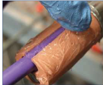
spread sealant over all external surfaces paying attention to joints.
