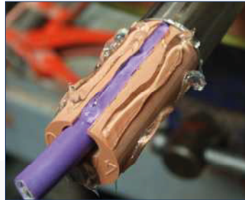
Apply sealant to outside of Lycron Block.
