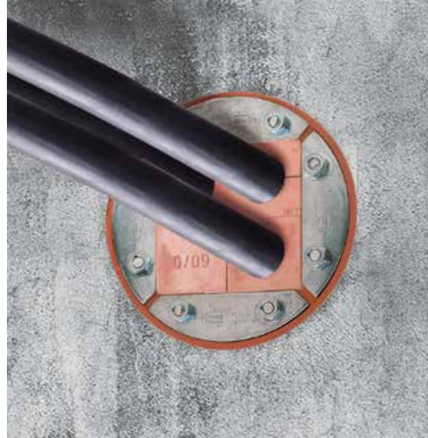
RGP transit placed in a drilled hole. No compression plate or final seal is required
