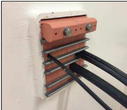
Push in the PTG into the frame. Make sure the PTG is placed inside the front and back edge of the stay plate.
