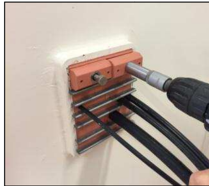
Tighten the two bolts evenly in steps.
