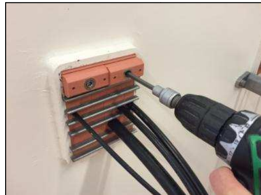
Tighten the two bolts evenly in steps.
